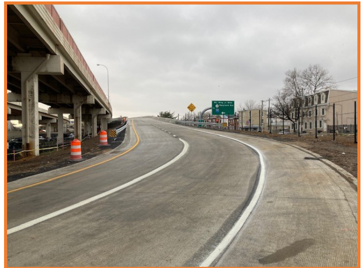
The new 2 nd Street on-ramp to I-95 southbound in Wilmington opened on December 31, 2020
